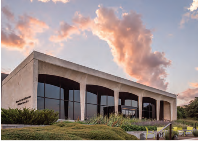
Fig. 4.22 Amon Carter Museum of American Art, Fort Worth, Texas, Philip Johnson (1906–2005), architect.
